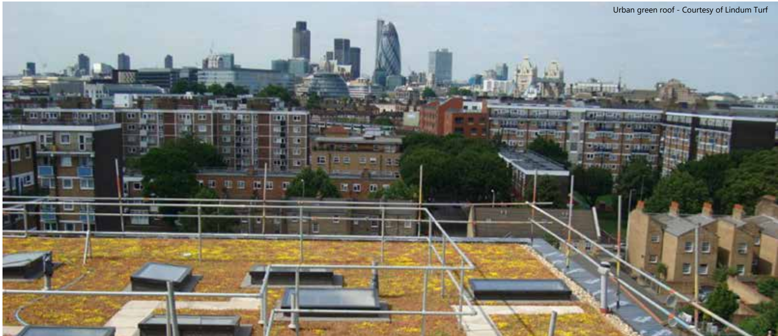
Urban green roof - Courtesy of Lindum Turf
